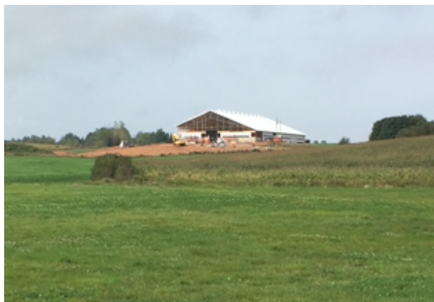
New McCurdy barn under construction
