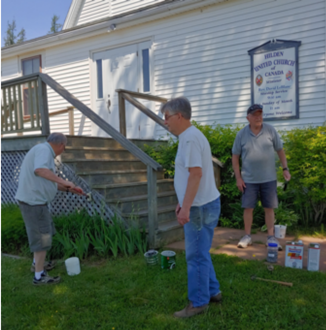
Painters at work.
